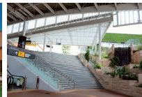
Minami-machida Grandberry Park Station
