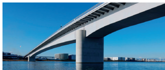
Tamagawa Sky Bridge
